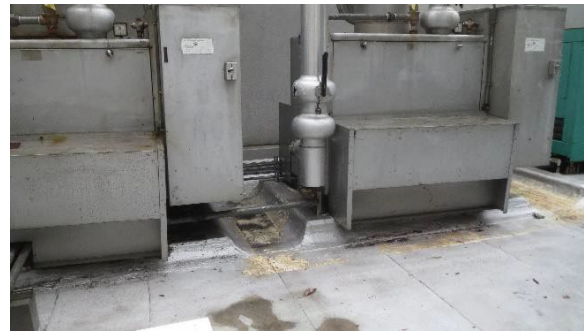
View boilers set on the roof pad.
